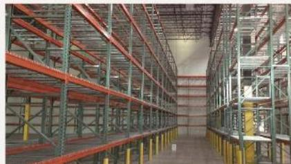
Gulf S. bolted frame consists of two uprights, horizontal and diagonal bracings, with bolted on or welded foot plates and adjustable at 2" height. Its available in a variety of sizes made it to be more flexible.
