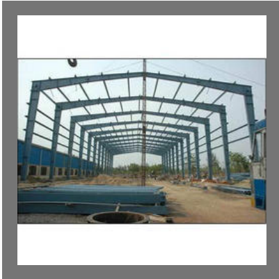
Pre Engineered Building Structure
